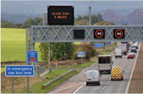
In normal operation, the bus lane is open and is indicated by a blank signal. Note the presence of an emergency refuge area.
