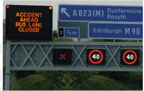
In emergency situations, the motorway signal over the bus lane is used to advise bus drivers that the bus lane is closed – a red 'X' signal is displayed over the bus lane and the variable message sign reinforces this.
