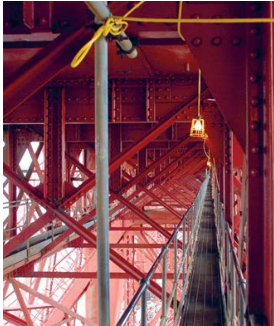
Detail of the access walkway and structural steel work beneath the permanent way in the south viaduct of the Forth Bridge, July 2011. (© Crown Copyright, reproduced courtesy of Historic Scotland. www.historicscotlandimages.gov.uk Miles Oglethorpe)
