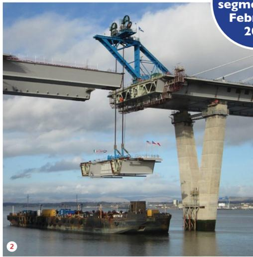
**2** A "fitting" conclusion: the final deck segment, weighing 570 tonnes, makes its way up to its destination. **3** Slipping neatly into the tight space at the top, members of the team can relax after another successful lift operation.
