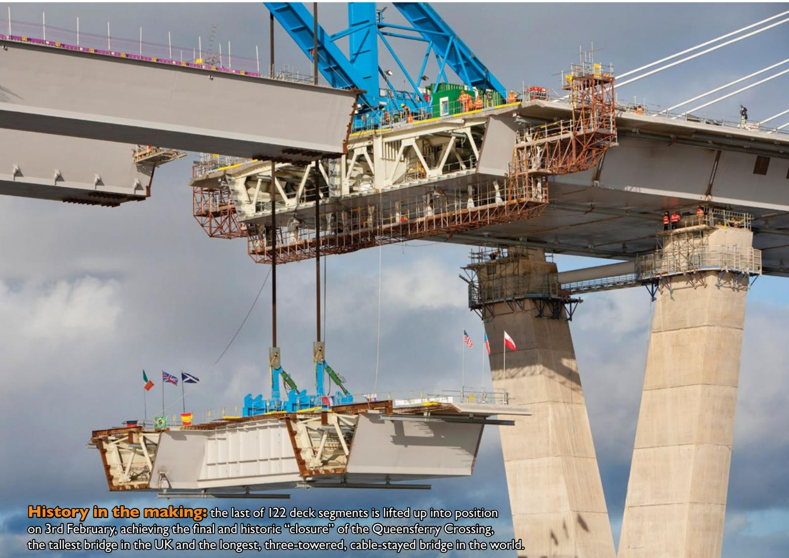
**History in the making:** the last of 122 deck segments is lifted up into position on 3rd February, achieving the final and historic “closure” of the Queensferry Crossing, the tallest bridge in the UK and the longest, three-towered, cable-stayed bridge in the world.
